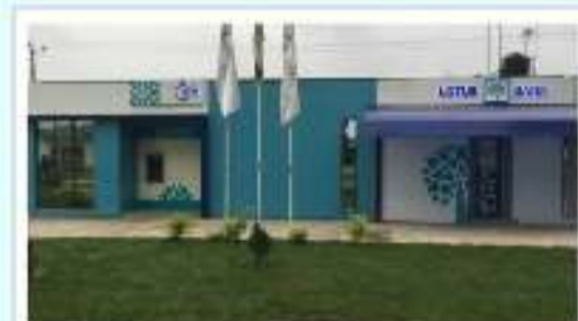
📍 Fountain University Campus, Oke-Osun, Osogbo, Osun State. 15th September, 2023
